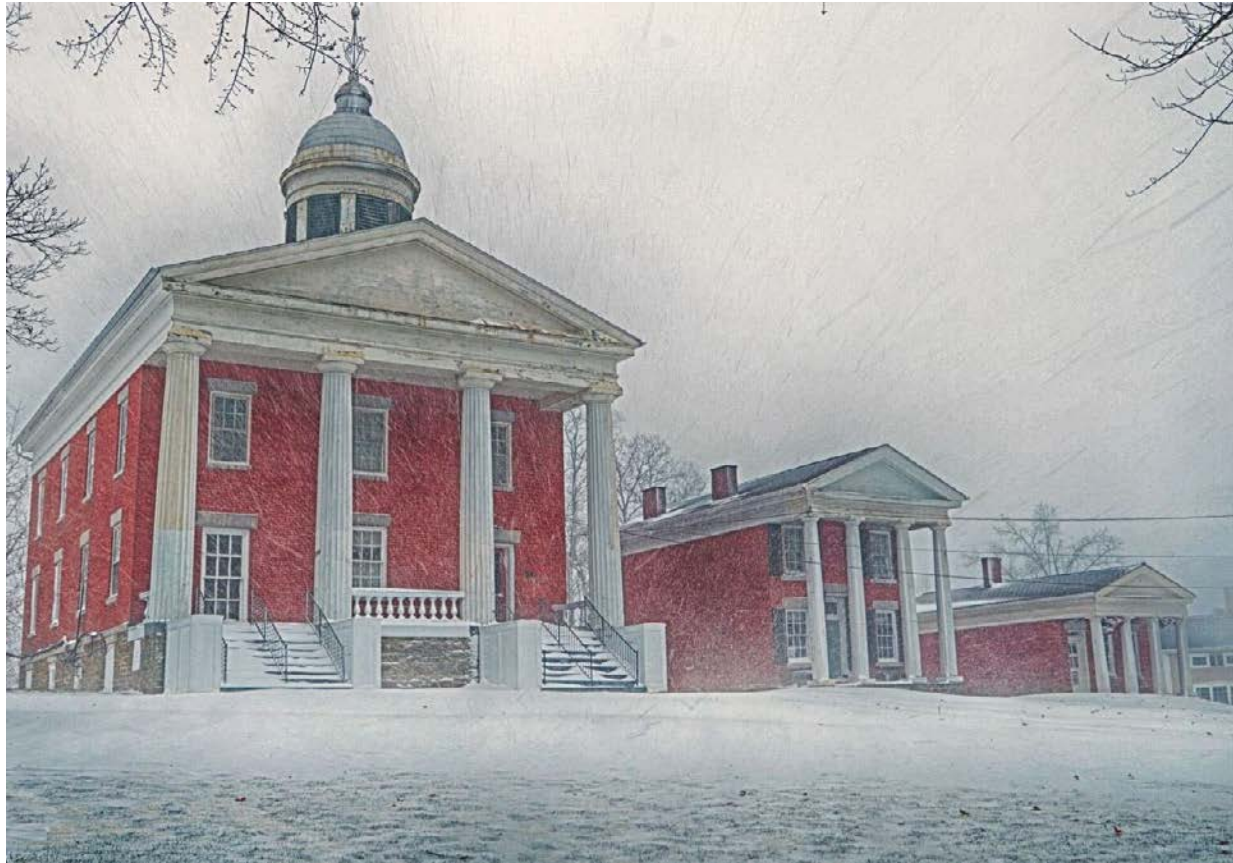
Photo 9. Ovid Three Bears is owned by Seneca County, cared for by Friends of Three Bears, and was named to the National Register of Historic Places in 1977. Photo by Carrie Smalser.
